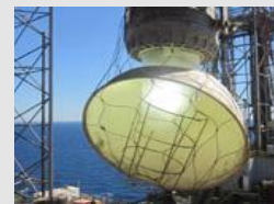
Light shade and impact guard dislodged due to corrosion
